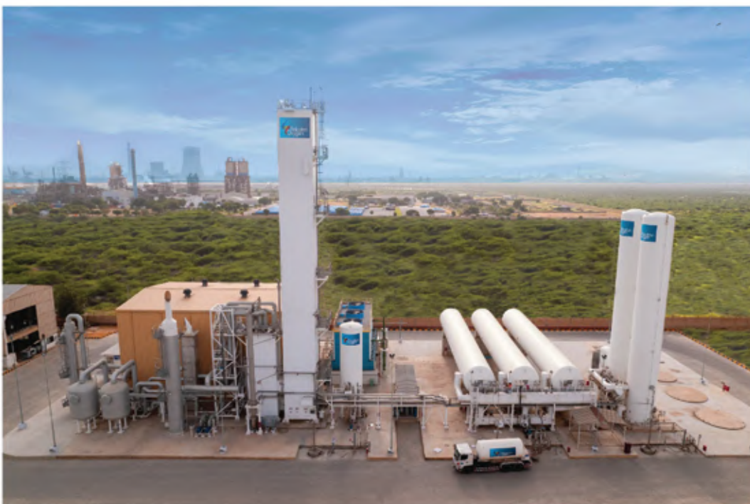
Country's largest 270 TPD Air Separation Unit plant at Port Qasim.
